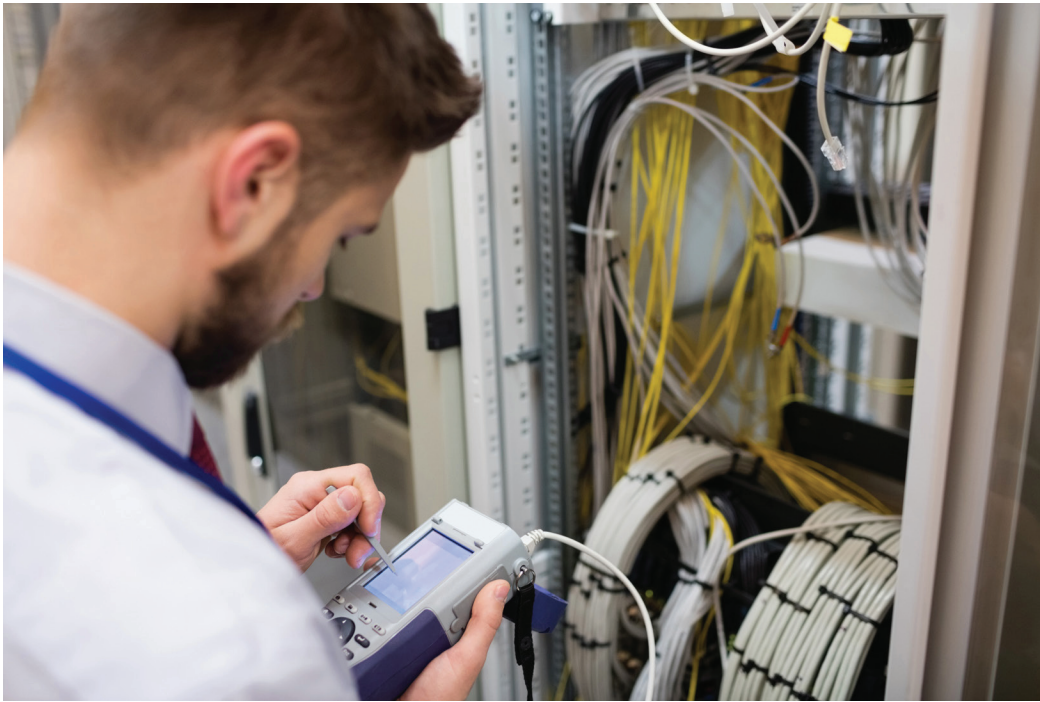
Technician using a cable certifier. (Image by Wavebreak Media © 123RF.com.)
